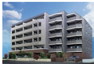
WAKOHRE Shinkobe Station Livlia Chuo-ku, Kobe-shi; a total of 33 units 6-minute walk from “Shin-Kobe” Station on Kobe City Subway To be delivered in November 2019
