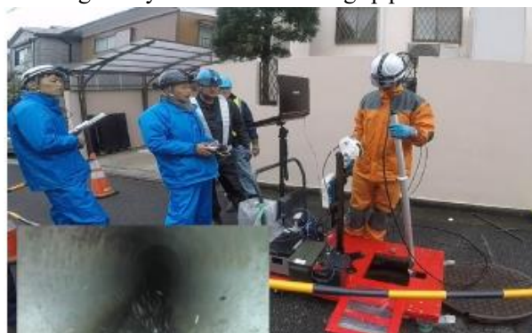
Screening survey of sewer and drainage pipes
