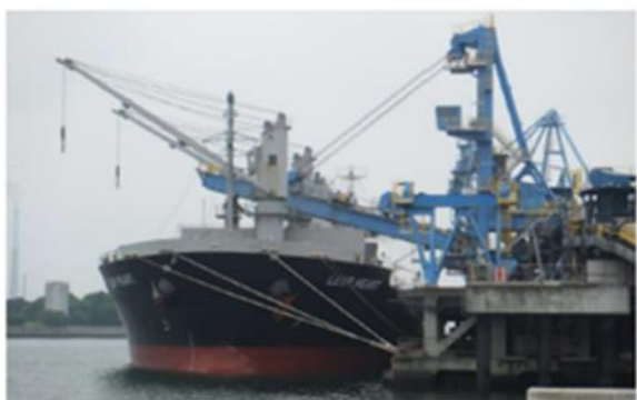
Clinker ship loader (Tokuyama Factory)
