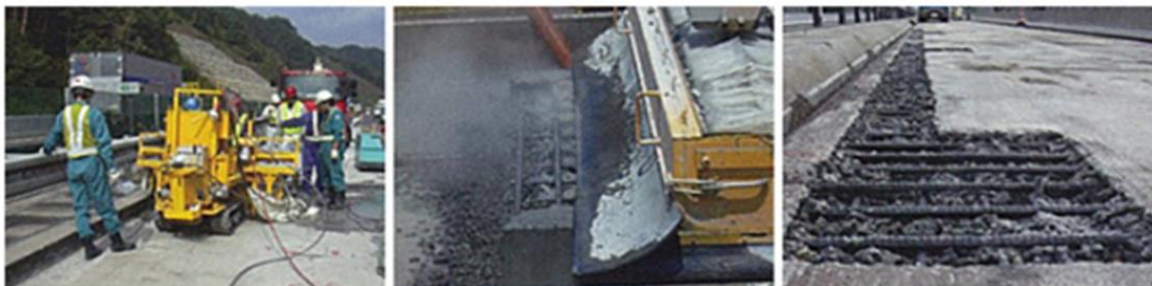
Removal of the deteriorated concrete floor slab suffering from salt damage
