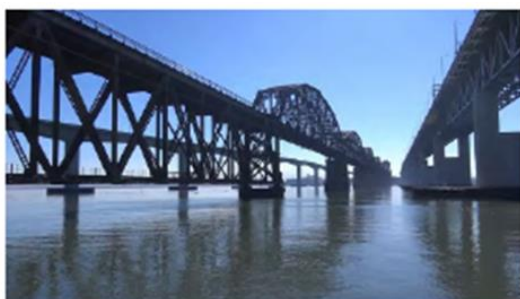
Inspection, etc. of steel-framed bridges (Source: AutoModality, Inc.)
