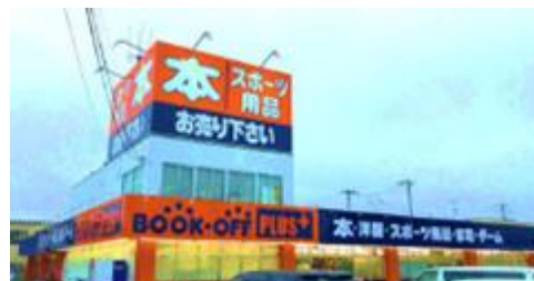
Route 50 Mito Motoyoshida Store: Exterior renovations
