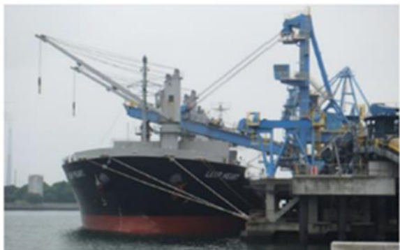
Clinker ship loader (Tokuyama Factory)
