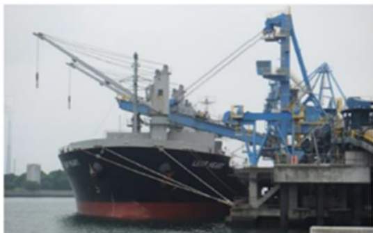
Clinker ship loader (Tokuyama Factory)
