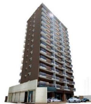
WAKOHRE Ikeda Station Flats 【Ikeda-City Osaka Prefecture】 (delivered in August 2020) 39 units in total. 4-minute walk from “Ikeda” Station on Hankyu Takarazuka line.
