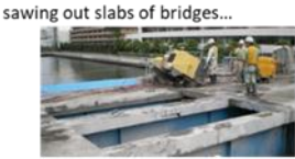
renewing bridges with remaining beams
