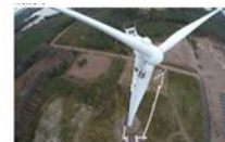
Used in the maintenance and upkeep of wind power generation facilities
