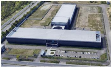
▲ Aerial view of Ishikari Data Center (front: Buildings 1 and 2, back: Building 3)
