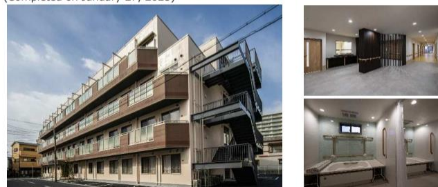
Renovation of Former Hospital in Abiko-Nishi, Sumiyoshi Ward, Osaka City (Completed on February 3, 2025)
