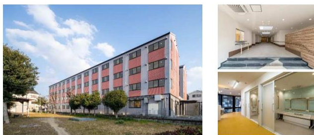
Renovation of Former Employee Dormitory in Yakumo-Higashi-Town, Moriguchi City (Completed on January 27, 2025)
