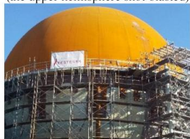
Shot-blasting machine Spherical gas holder (the upper hemisphere shot-blasted)
