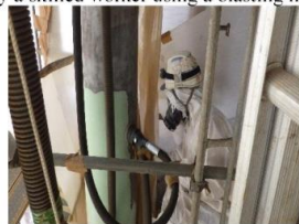
Scene of work with a machine Removal of the paint by a skilled worker using a blasting method
