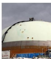
Scene of work with a machine Removal of the paint by a skilled worker using a blasting method
