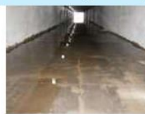
DUCTAL Panel Lining Method
