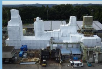
Curing sheet made of recycled plastic
