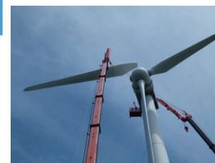
Blade disassembly
