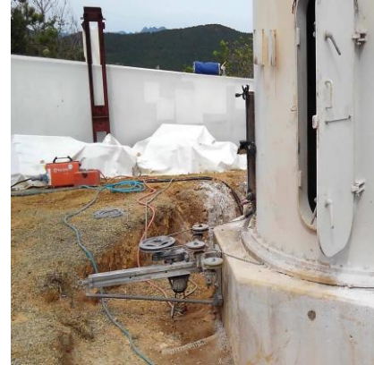
Wire sawing method
