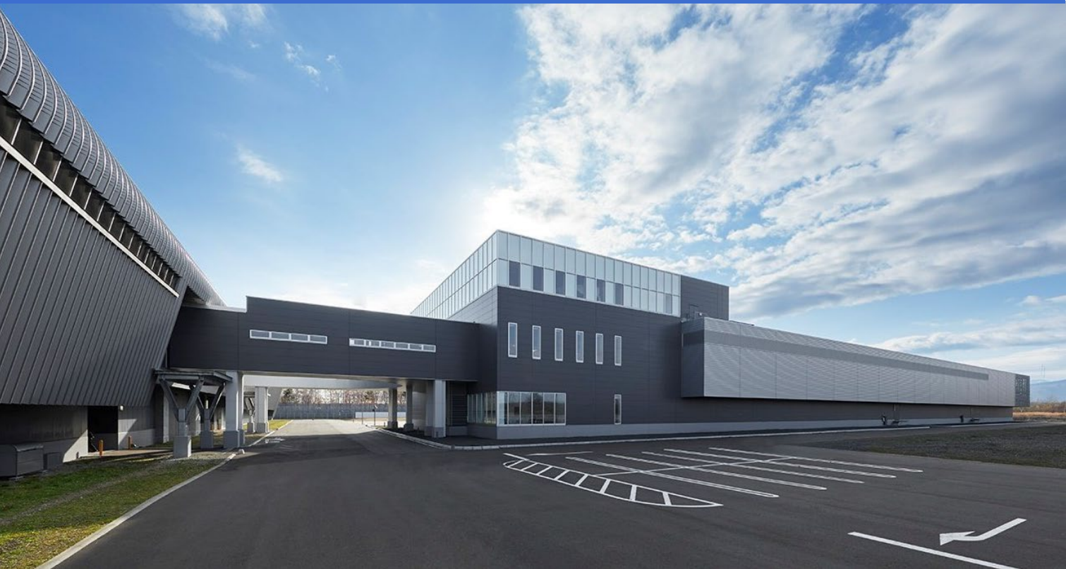
Building 3: Indirect outdoor-air cooling system
