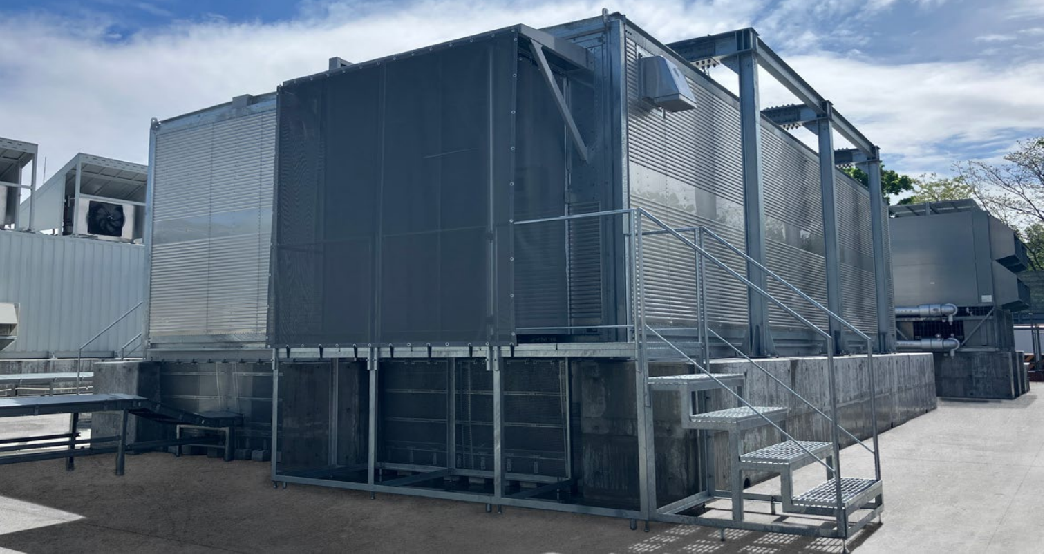
Container-type: Direct liquid cooling system (DLC system)
