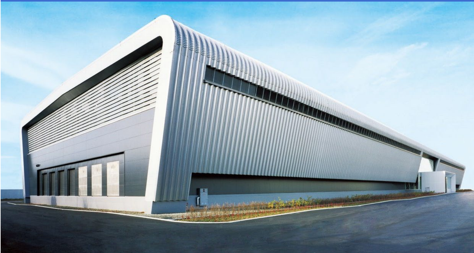
Buildings 1 and 2: Direct outdoor-air cooling system
