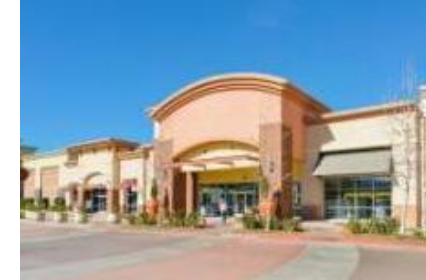
Commercial facilities /public facilities
