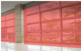
Glass wall protection
