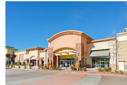
Commercial facilities /public facilities
