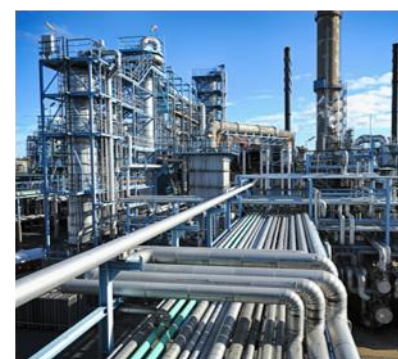
Oil, gas, and other infrastructure facilities
